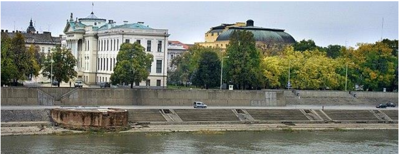
Tisza riverside with Móra Museum, and the National Theatre Szeged – building
